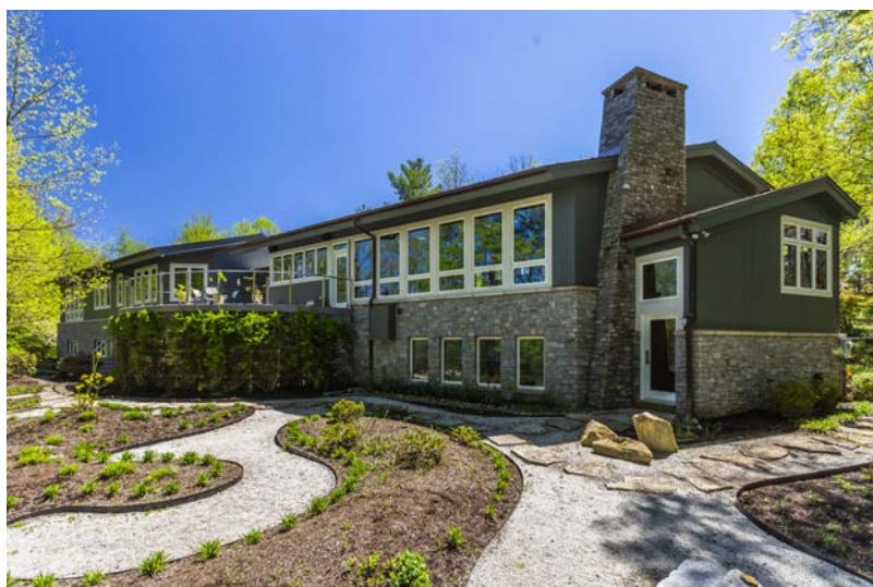
The exterior of the Smiths’ Lexington, Ky., home. PHOTO: MATT HUBER / MATT MEDIAWORKS
