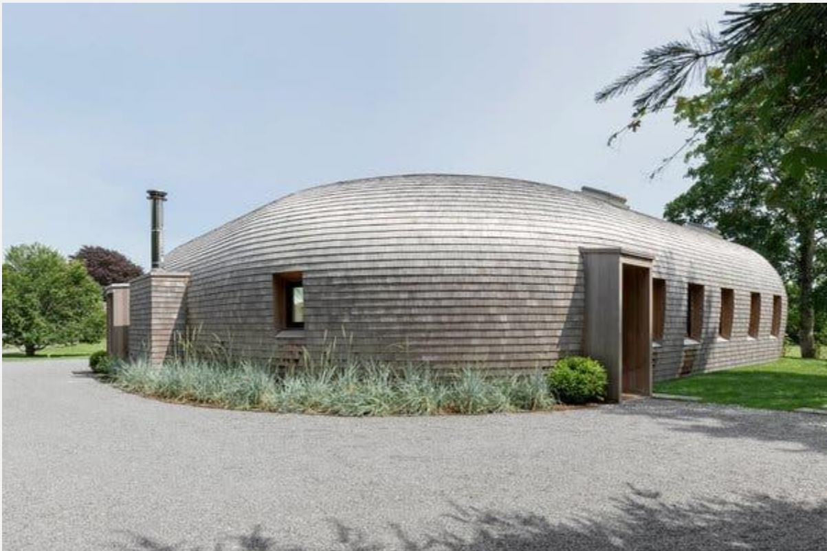
The thick and heavily insulated walls of the north and west sides hold the heat and offer privacy. Credit...Caylon Hackwith
